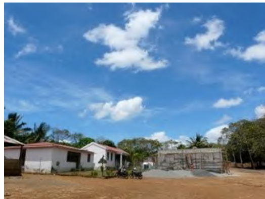
(Expansion of the Community Clinic)
